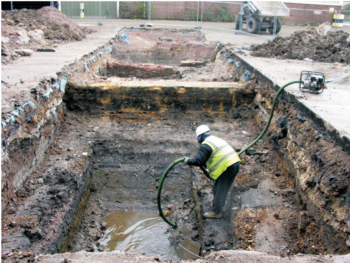
Fig 17 Trench 9, looking southeast
