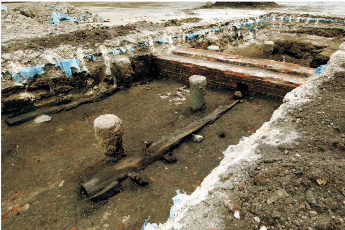
Fig 16 Small Mast Pond wall [402] and timber tie backs [431] and [429] in Trench 7, looking north
