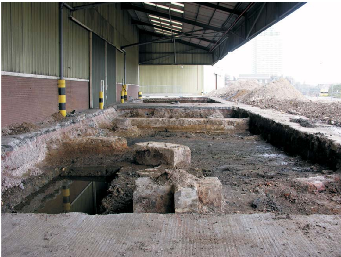
Fig 42 Trench 37, looking northwest
