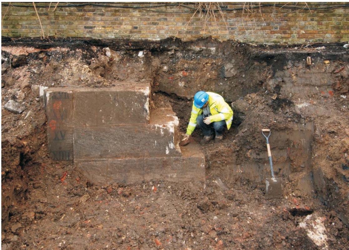
Fig 57 East wall [397] of the Great Dock in Trench 50, looking southeast. Painted depth gauge on left
