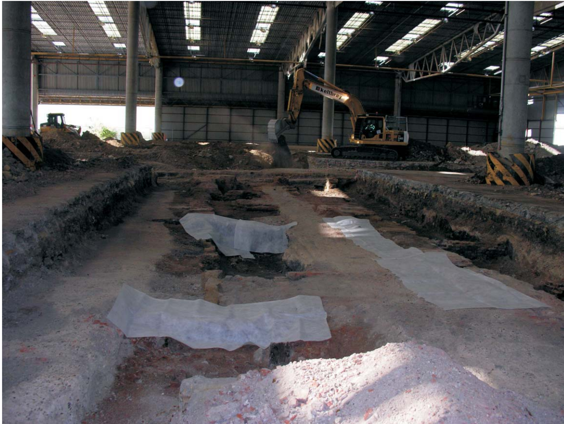
Fig 66 Backfilling Trench 47, looking southwest
