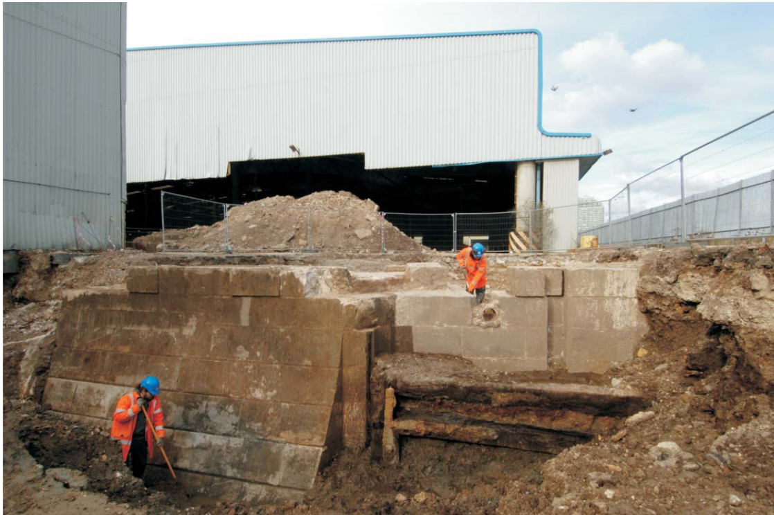
Fig 56 West wall [457] of the Great Dock in Trench 50, looking northwest. Iron and timber dock gate to right
