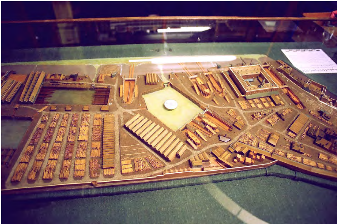
Fig 7 The 1774 model, looking 'north'. Dockyard Basin is in the centre of the image, the small mast pond to the west of this, storehouse complex to the east. Note the slipways and extensive areas used to stockpile timber
