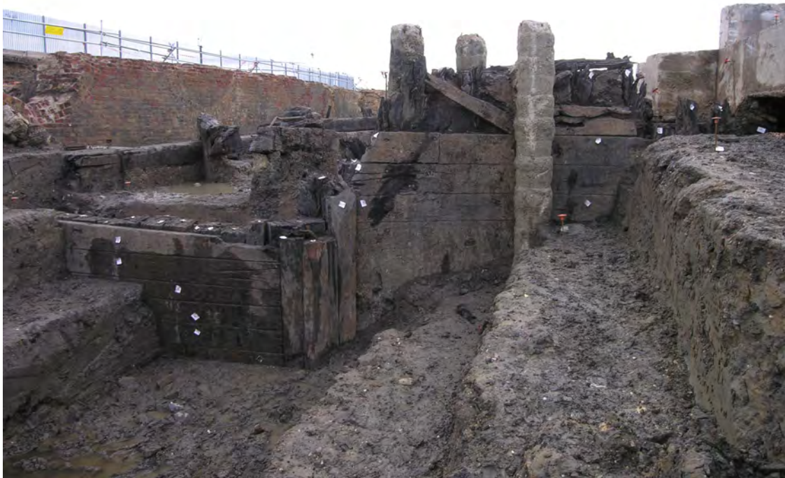
Fig 27 Timber basin gate with copper plate depth gauge in Area 2, looking east
