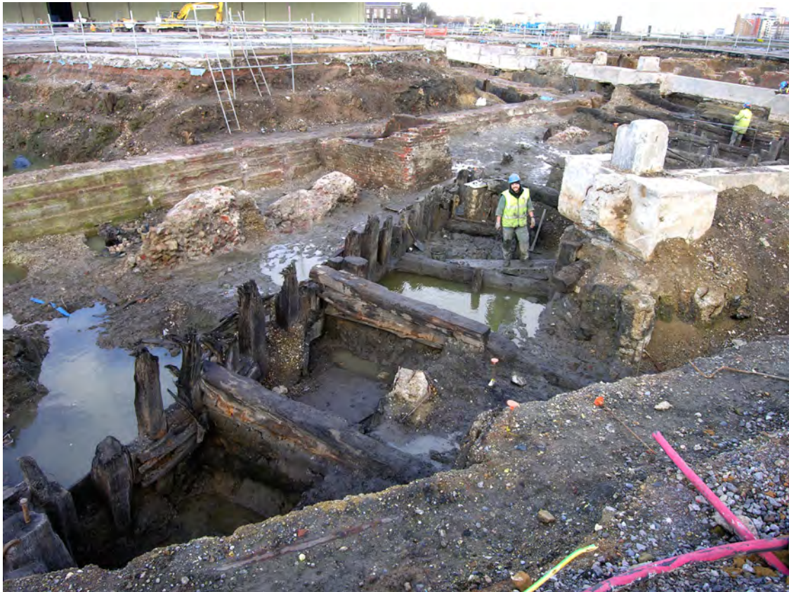
Fig 23 Eastern part of the timber basin wall with land ties and a brick crane base in Area 3, looking west
