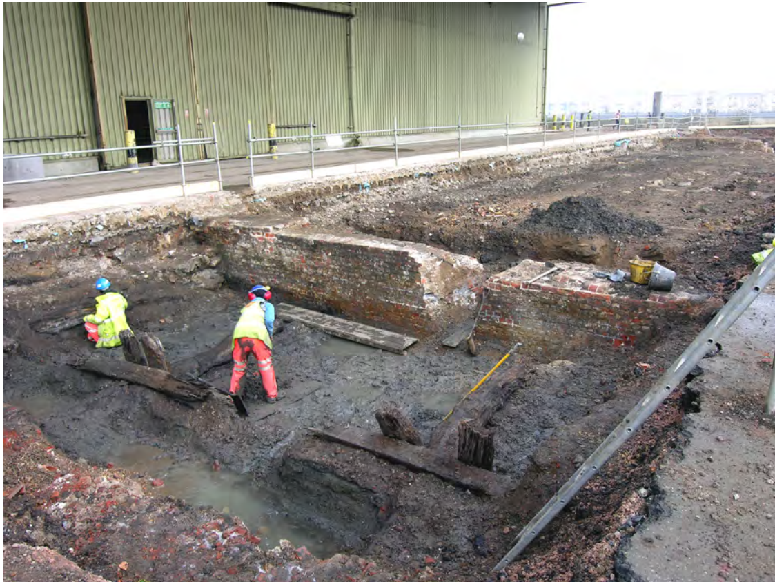
Fig 54 Small Mast Pond wall and tie backs in Area 1.2, looking northwest
