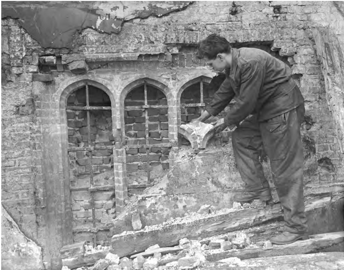
Fig 18 A four-light mullioned window of the Tudor storehouse revealed in 1952
