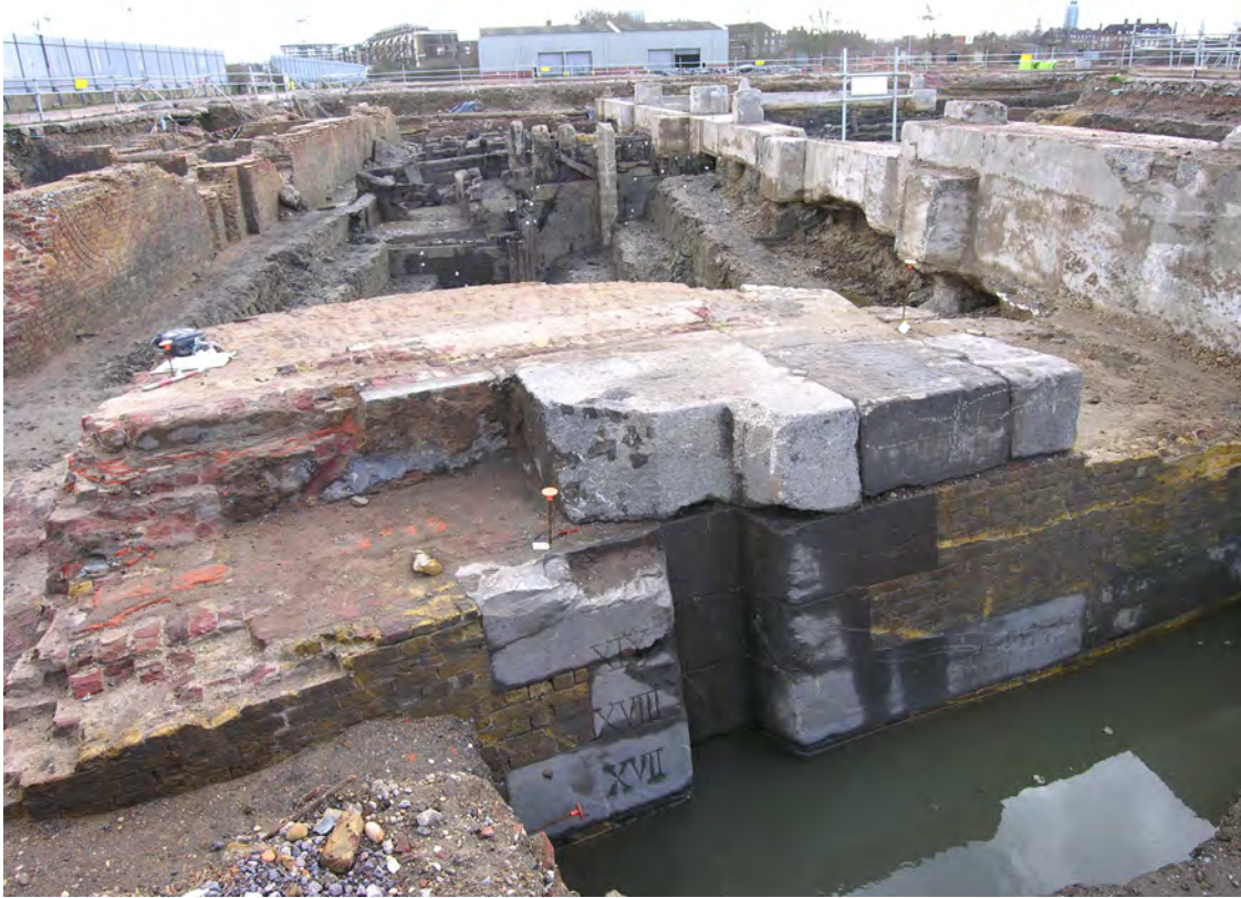
Fig 74 Eastern part of the brick basin gate with depth gauge (in Roman numerals), in Area 2, looking east. Note superseded earlier timber gate in background
