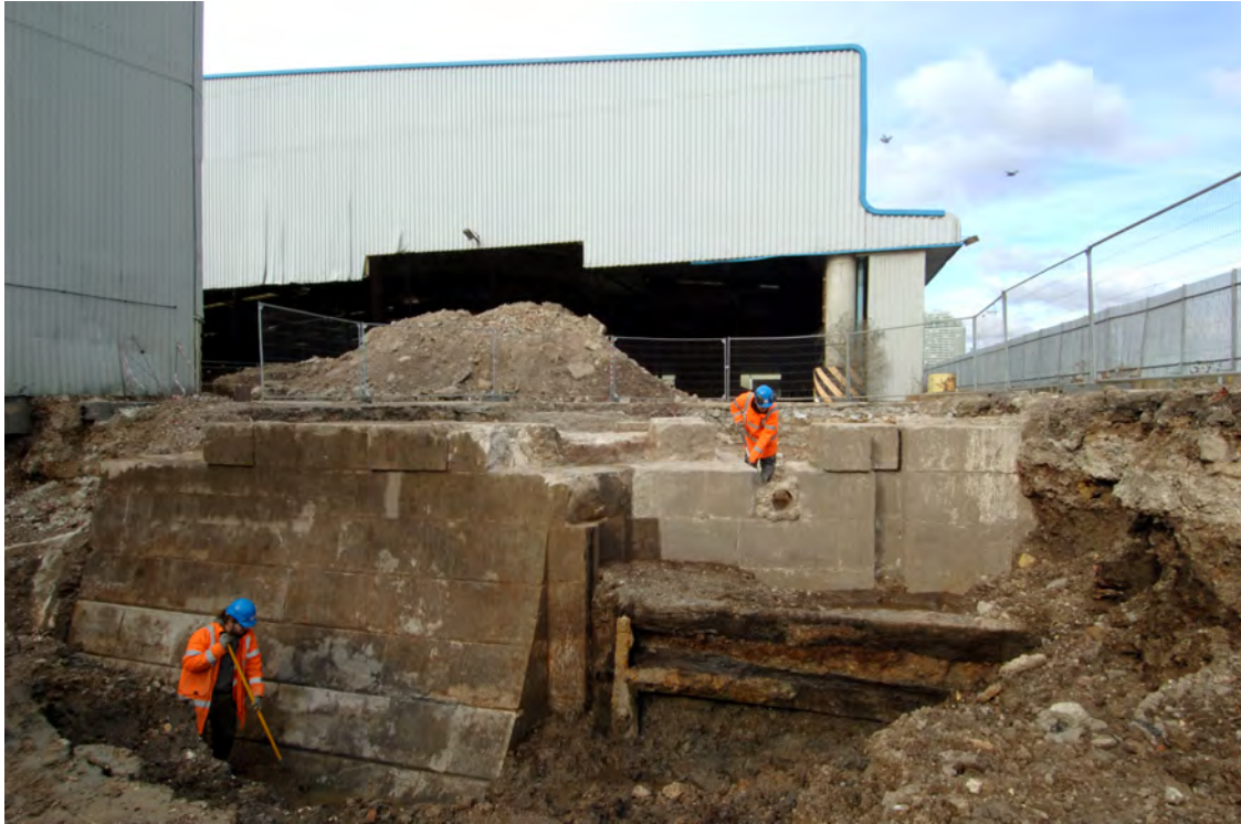
Fig 87 West wall of the Great Dock in Trench 50, looking northwest. Iron and timber dock gate to right
