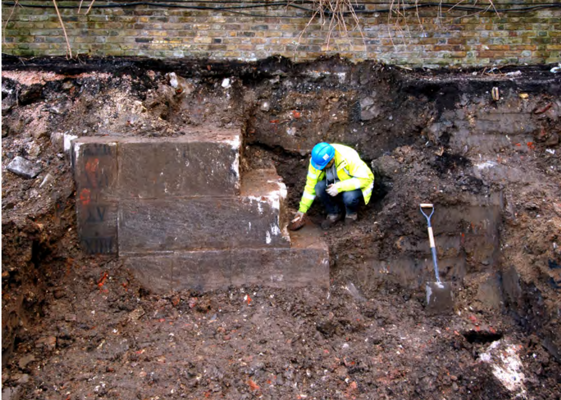
Fig 89 East wall of the Great Dock in Trench 50, looking southeast. Painted depth gauge on left
