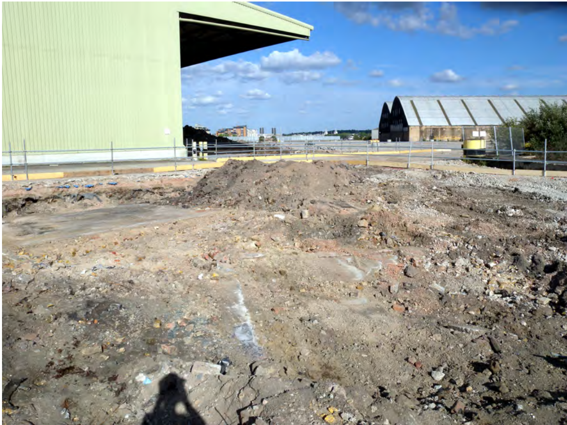
Fig 107 Areas 11 and 9 (in background), looking northeast
