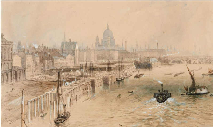
Construction of the embankment 1858, as part of Bazalgette's scheme. The Embankment incorporates the new sewage system for London and ultimately routes for the District and Circle Line.
